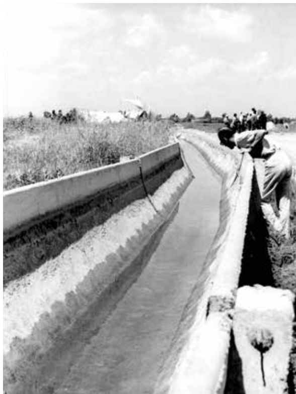
Figure 28. Monitoring and cleaning of the irrigation canals in Turkey, 1972
