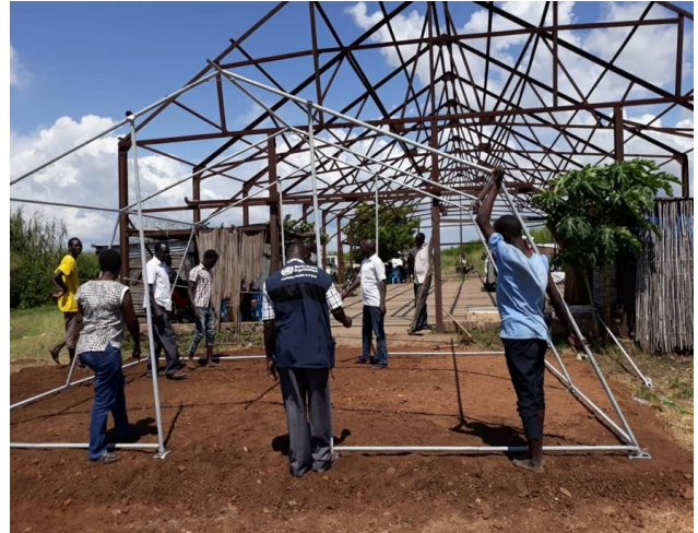
Construction of the Nimule River Port screening site. Photo: WHO
