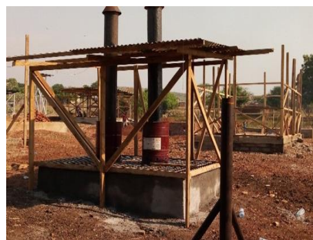
Ongoing construction of the isolation facility in Nimule
