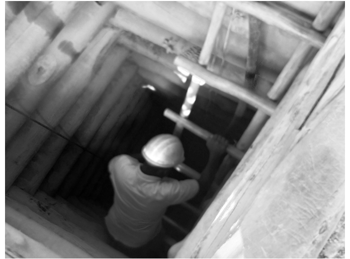
Figure 15: Mining pit with secured walls
