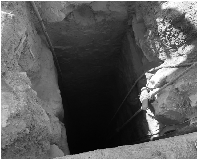
Figure 14: Mining pit with unsecured walls
